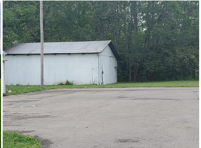
Existing Accessory Structure
