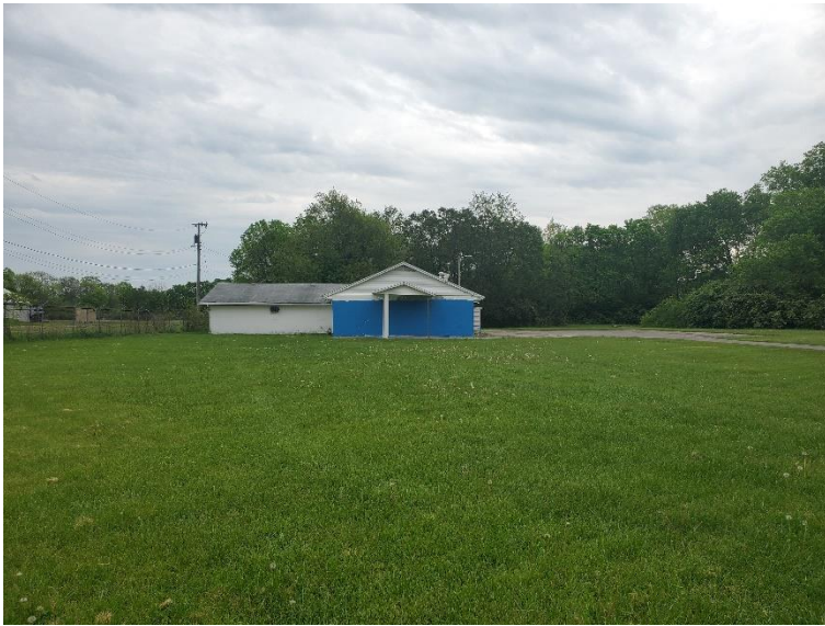
Front of Subject Site
