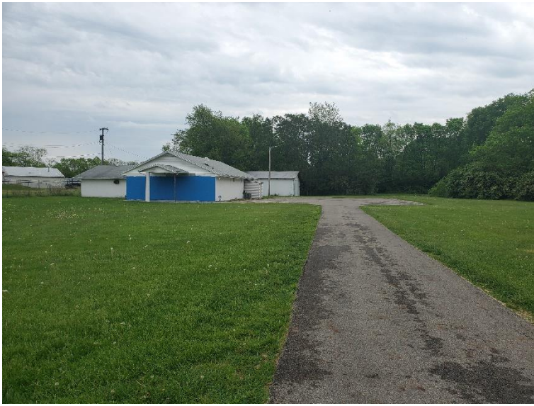
Principal Structure (former Church)
