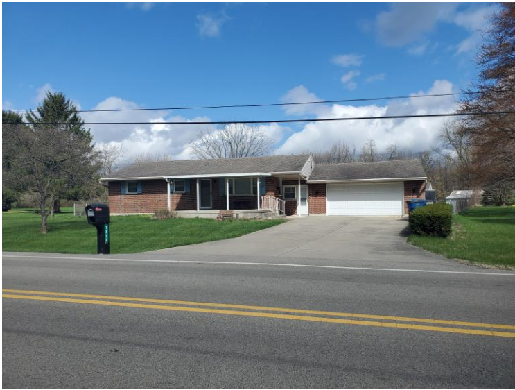
Front of Subject Site
