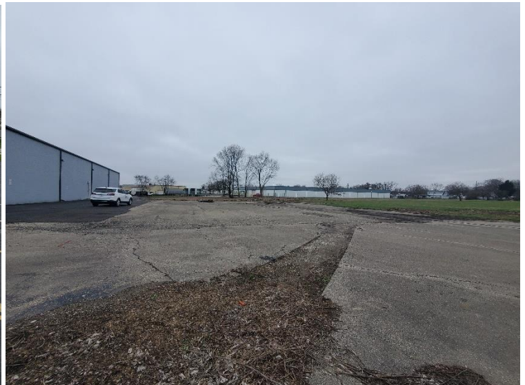
Rear of Subject Site
