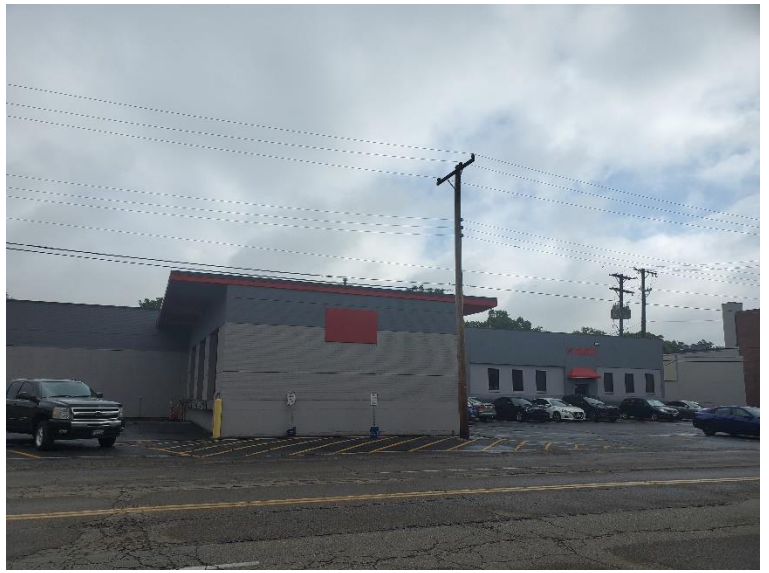
Adjacent Property Across Springfield Street
