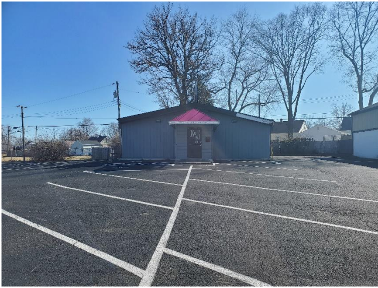
Front of Subject Site
