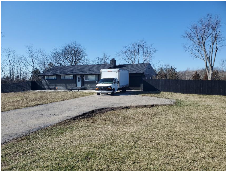
Front of Subject Site
