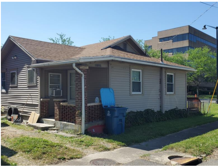
Front of Subject Site
