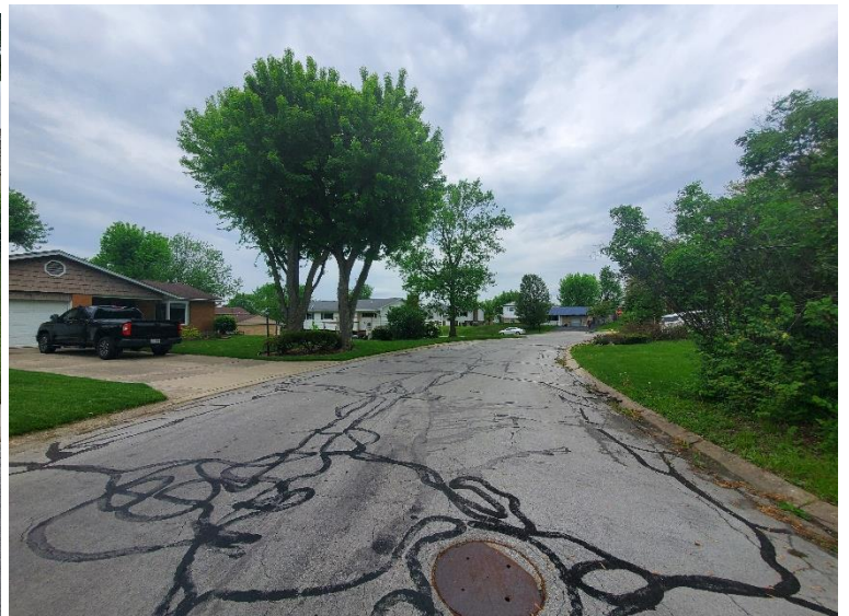
Adjacent Properties to the South
