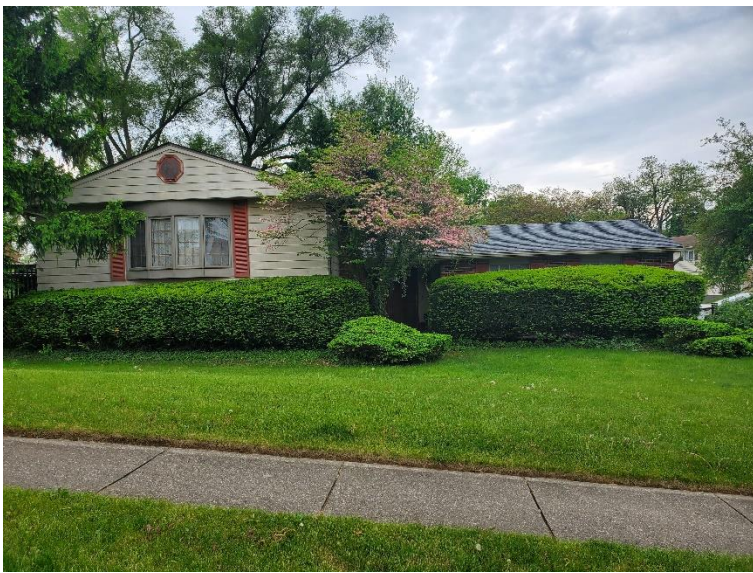
Front of Subject Site
