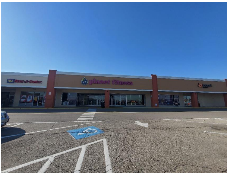
Front of Subject Site
